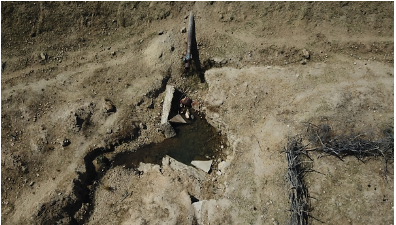
Irrigation outlet pipe and non-existent valve chamber
