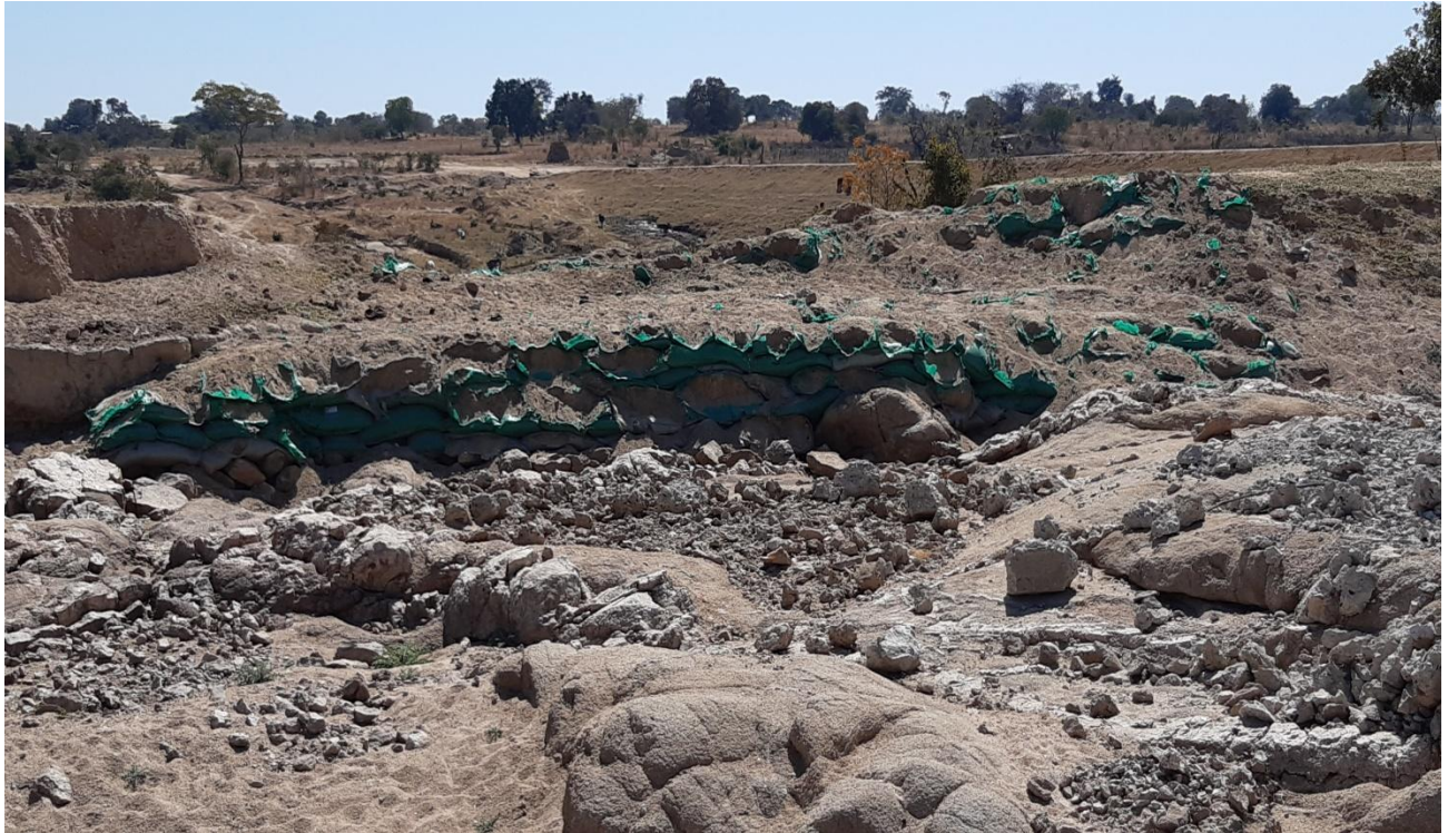
Figure 22 Spillway and causeway erosion; along drop structures- eroded areas and failed drop weirs 1
