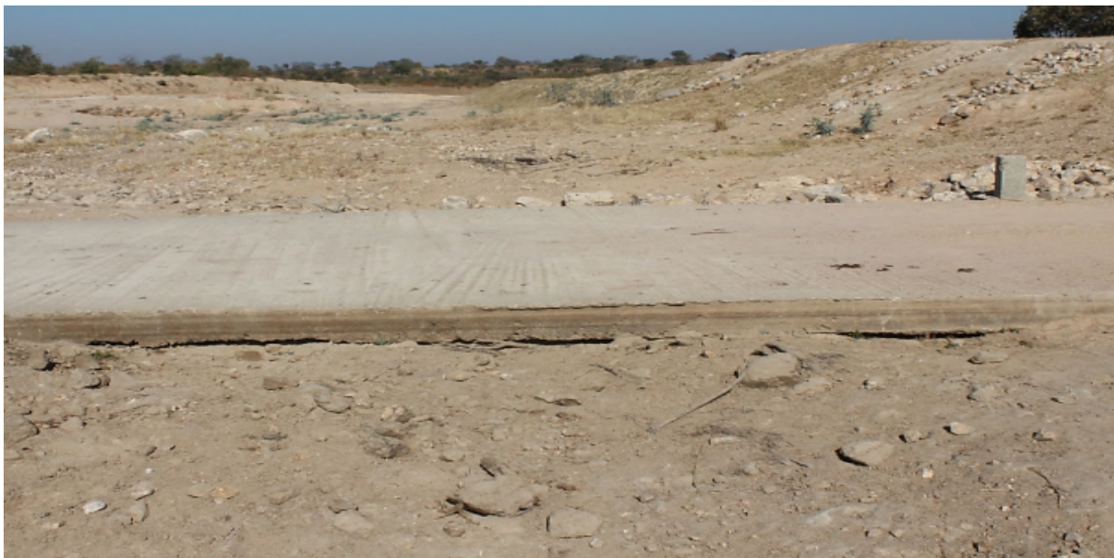
Figure 45 Causeway undercutting, access safety risk
