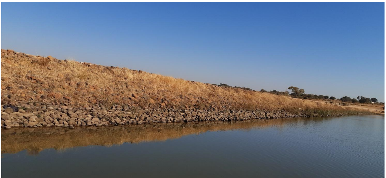
Figure 4 Stone pitched and grassed upstream embankment
