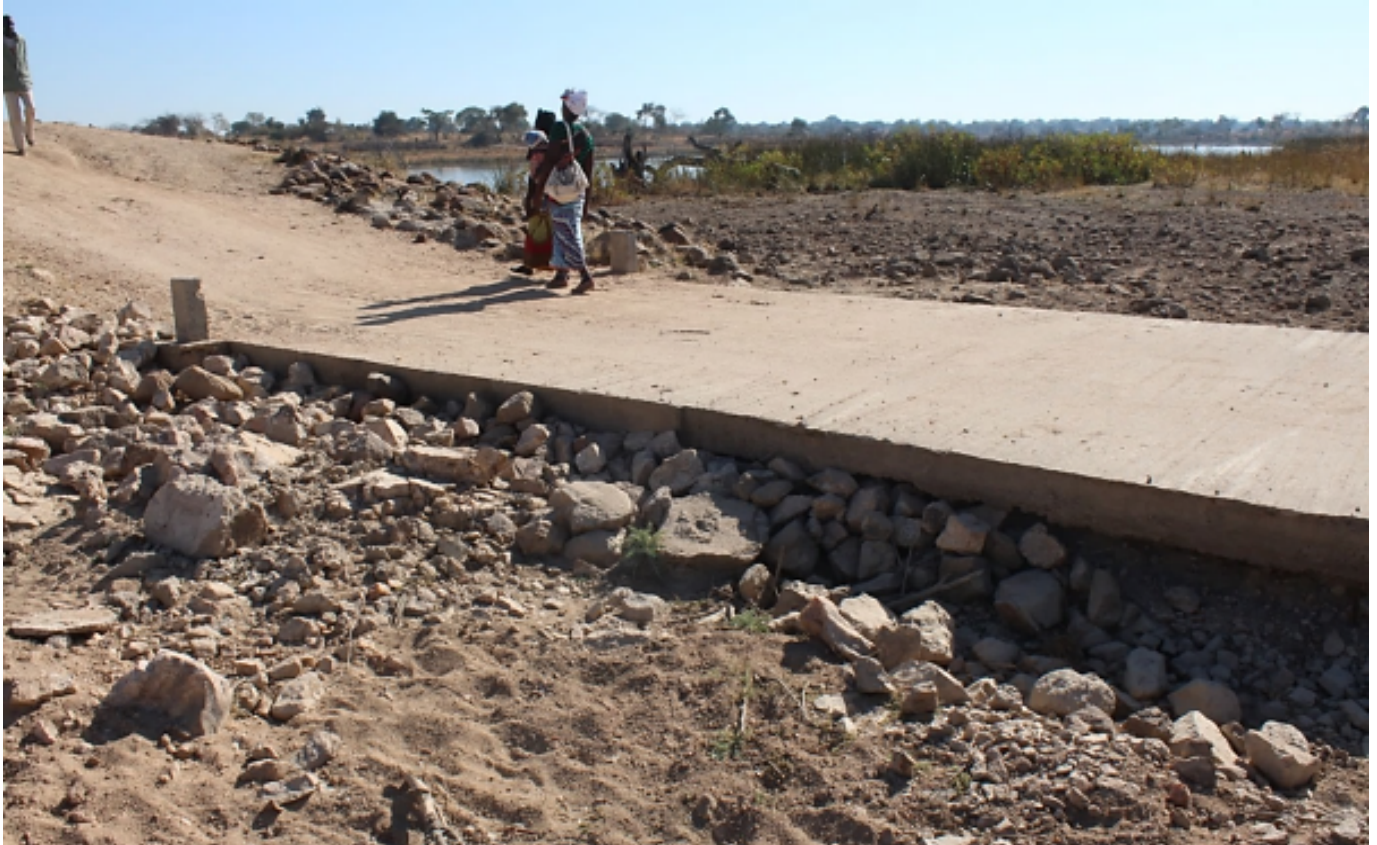
Right hand end of causeway from downstream showing undercutting
