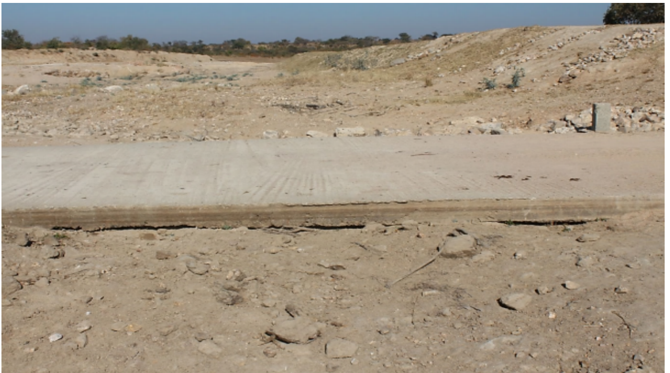
Spillway undercutting viewed from upstream – no cut off constructed
