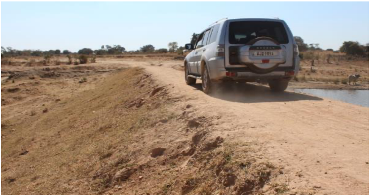
Figure 21 Narrow crest access road, also showing signs of erosion
