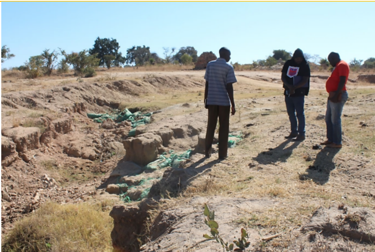
Secondary spillway gully and temporary repairs from 2018
