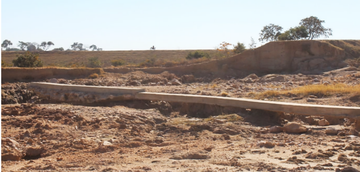
Figure 46 Drop structure complete washout and undercutting, dam safety risk
