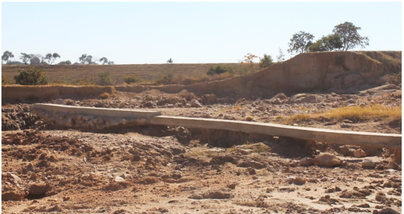
Drop structure complete washout and undercutting
