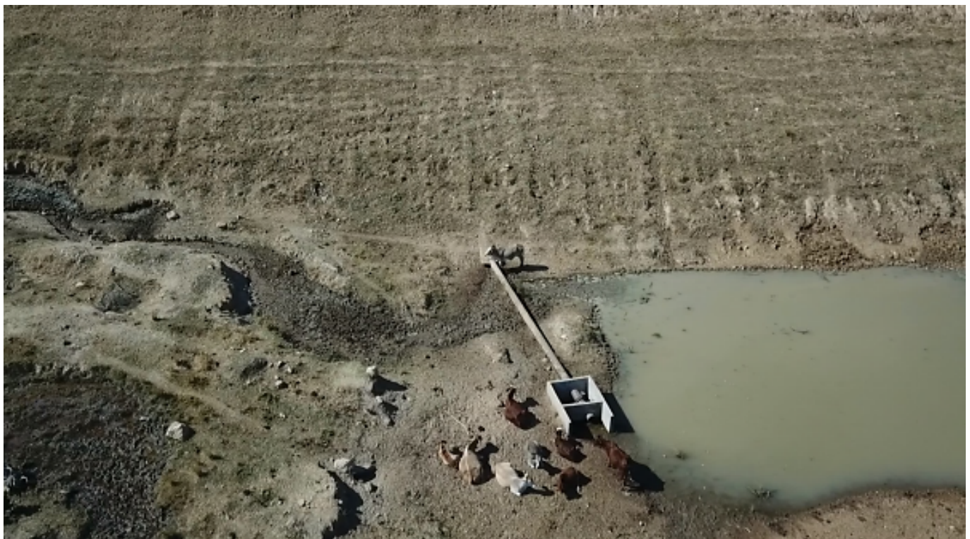
Low flow pipe and valve chamber and apparent lateral movement
