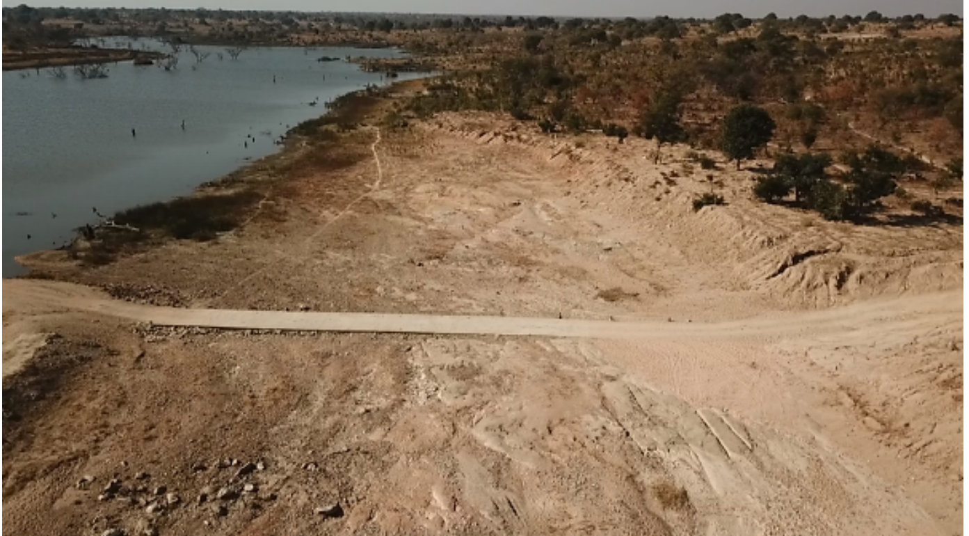
Inlet channel to spillway sill and causeway
