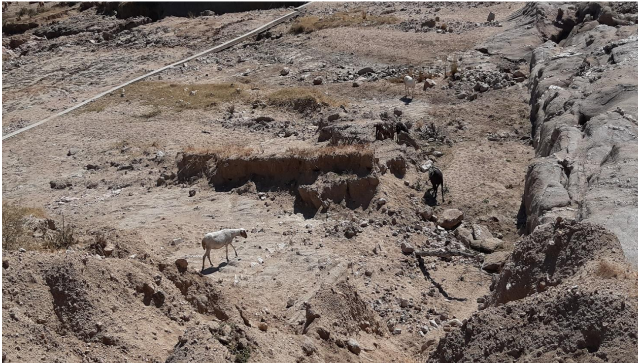
Figure 23 Spillway and causeway erosion; along drop structures- eroded areas and failed drop weirs 2
