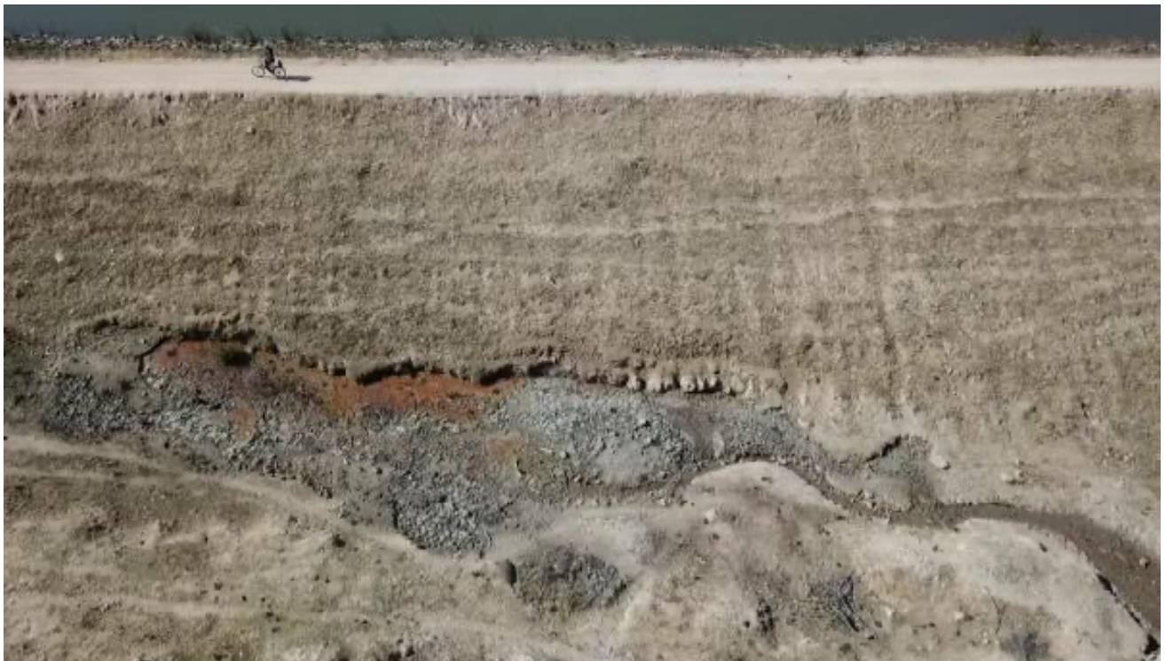
Figure 19 Downstream of the embankment showing soil loss
