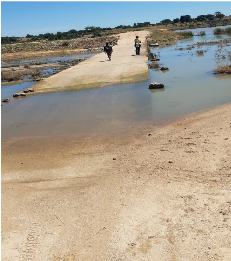
Figure 29 Flooded causeway access point, March 2021
